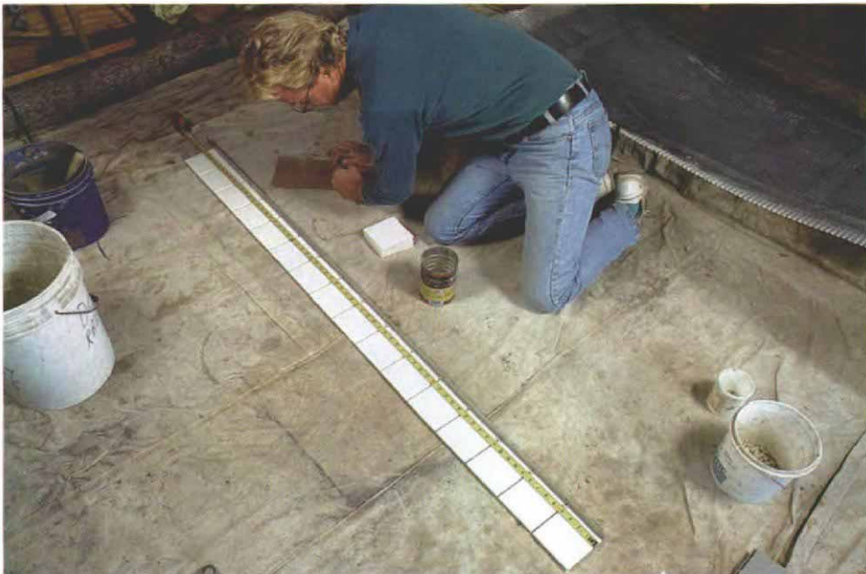
Measure the tiles. To plan tile cuts, space a row of tiles along a straightedge, measure the distance from the end of the row to each joint and correlate the measurements with actual wall dimensions.
