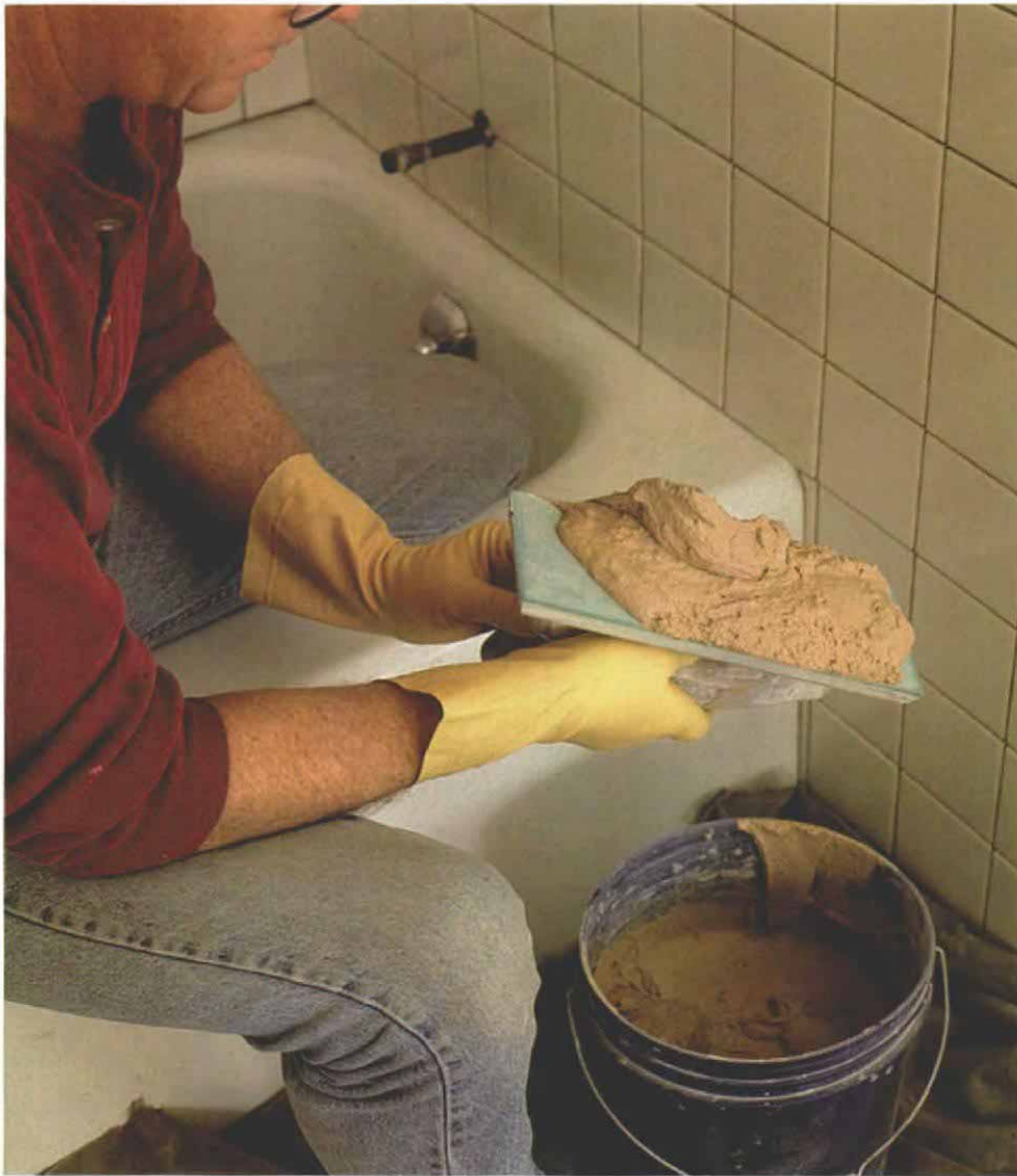
Ready for grout. Load freshly mixed grout onto the rubber face of a grout trowel.
