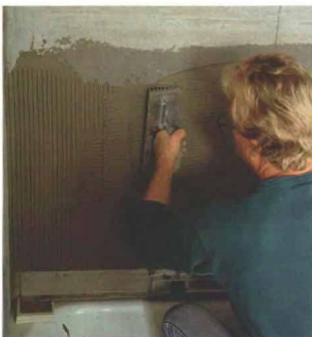
Spreading mortar. Use the straight edge of the notched trowel to spread thin-set mortar. Use the notched edge to comb uniform ridges.
